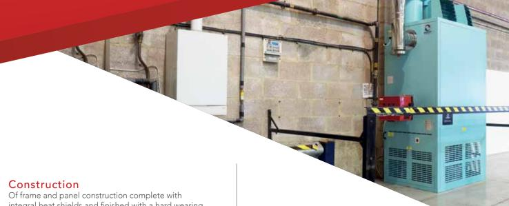
Of frame and panel construction complete with integral heat shields and finished with a hard wearing epoxy powder coat stove baked paint.
